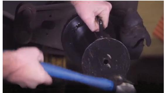
Drive seal onto spindle
